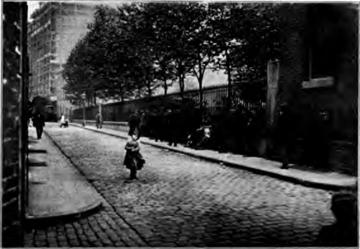
THE LINE WAITING BEFORE WHITECHAPEL WORKHOUSE.
